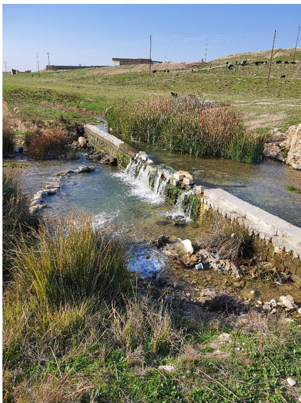
D4-3 Weir on the west spring for diversion water
